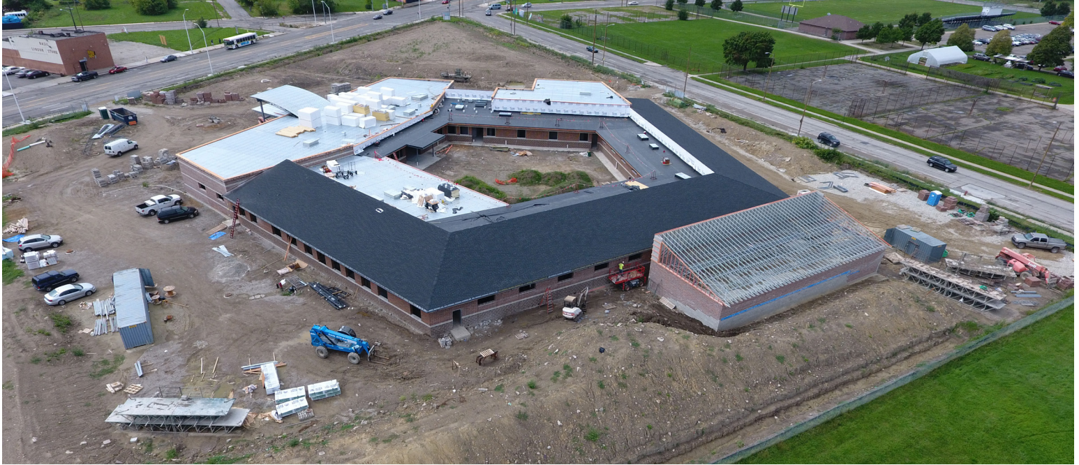
Drone photos courtesy of L.S. Brinker
