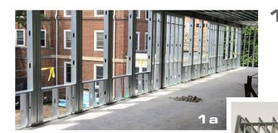
At the new University of Michigan William Monroe Trotter Building, Stenco teams have installed cold form metal framing for the exterior walls and roof. The team is currently completing the building enclosure and will continue on with the interior package in the coming weeks, including walls, ceilings, wall protection, and accessories. The project is on schedule to be completed in February of 2019.
