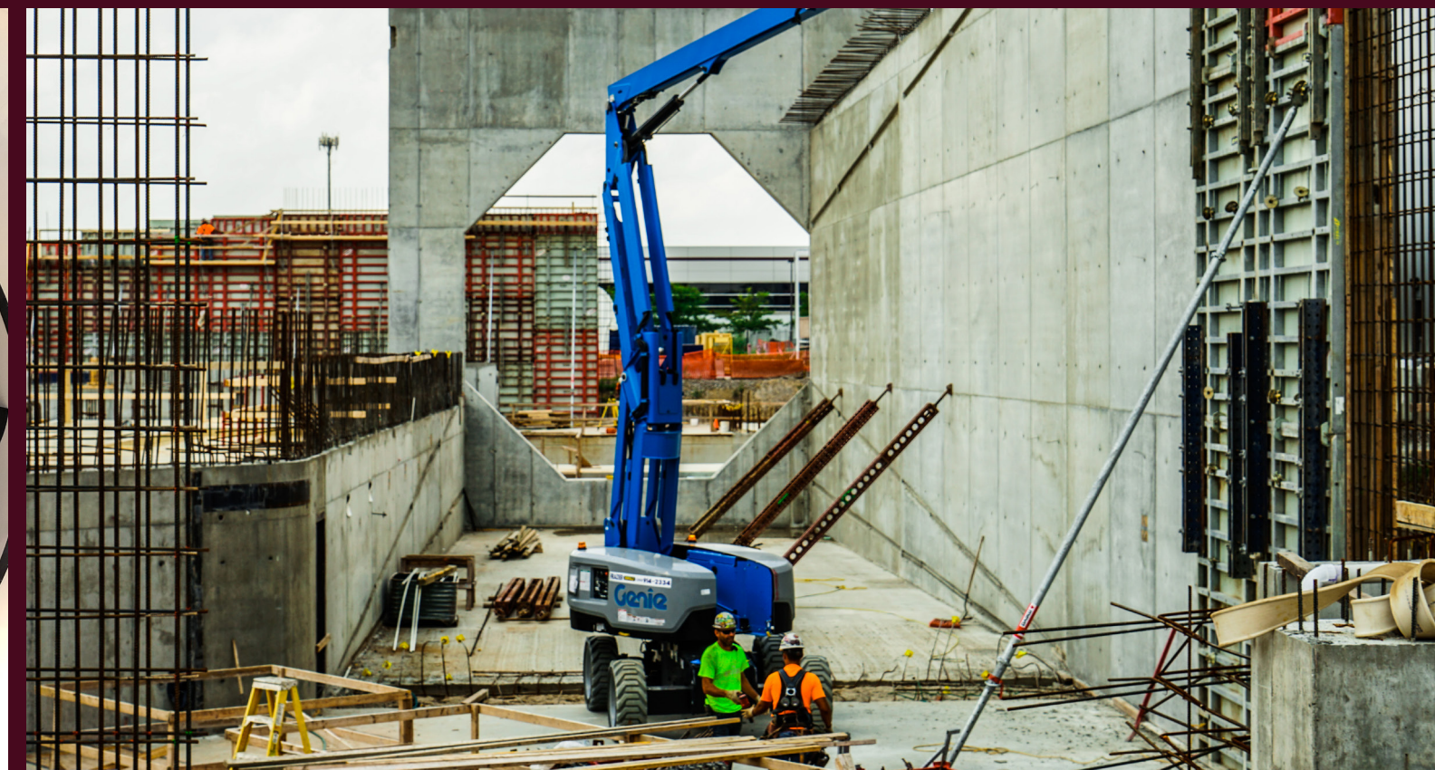
The wind tunnel fan sits in a 28-foot-tall concrete octagon box-out.
